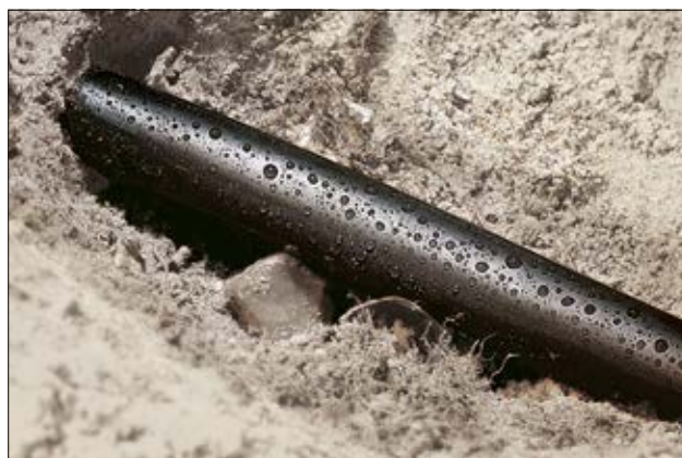
TREDUX HA47 - application below ground.
